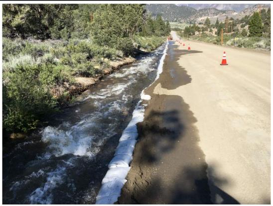
Photo 1 – Shoulder Erosion Undercutting asphalt Edge – View West
