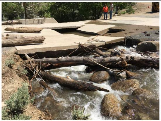
Photo 3 – Failed Up-stream Headwall and Debris – View North-East
