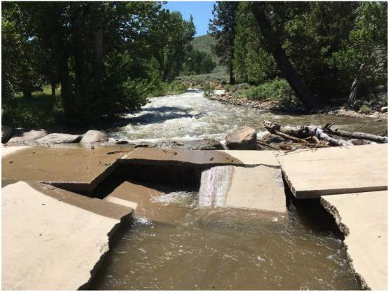
Photo 2 – Culvert Backfill Material Completely Eroded Under Slab – View South
