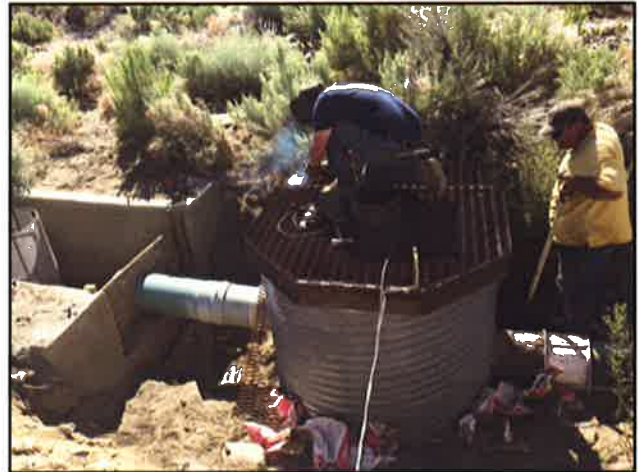
Installation of a self-cleaning irrigation water filter at Cinnamon Ranch.
