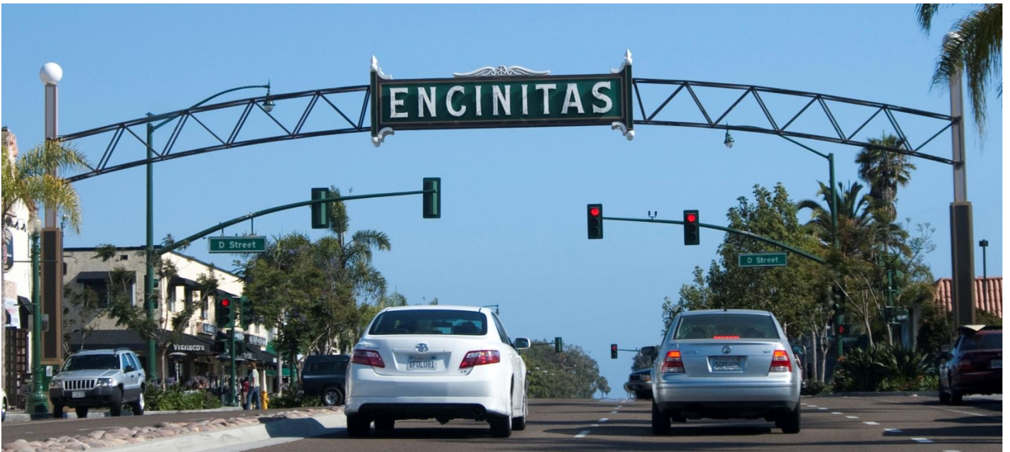
Encinitas CA Arch: Crosses State Hwy 1, built in 2007, Span is 80-feet 0-inches.
