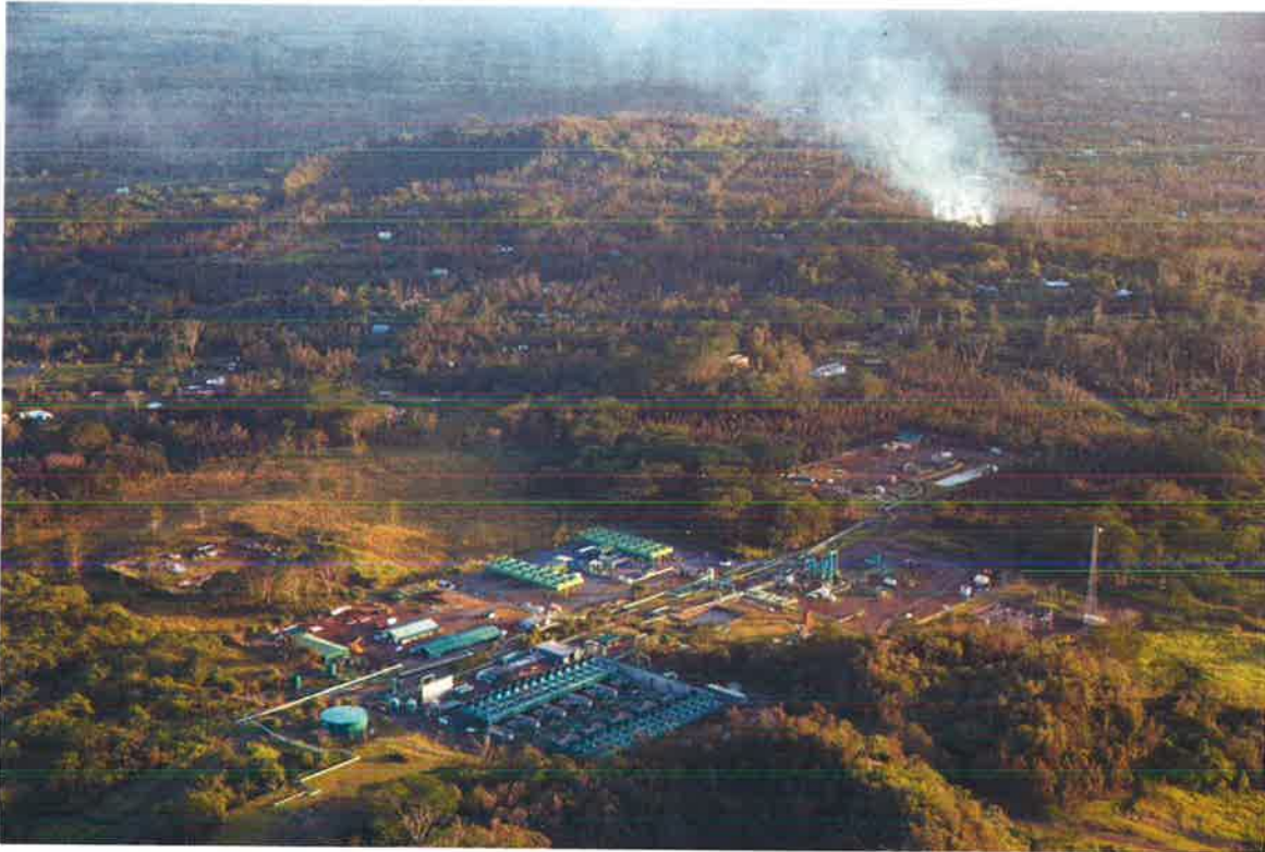
An aerial view of the Puna Geothermal Venture, a plant that lies just downslope of the erupting Kilauea volcano on Hawaii's Big Island. Smoke rises from the lava flow on May 4 as it made its way through the Leilani Estates subdivision near Pahoa. (Bruce Omori/Paradise Helicopters/EPA-EFE/Shutterstock)
