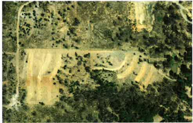
Unabated water run-off
