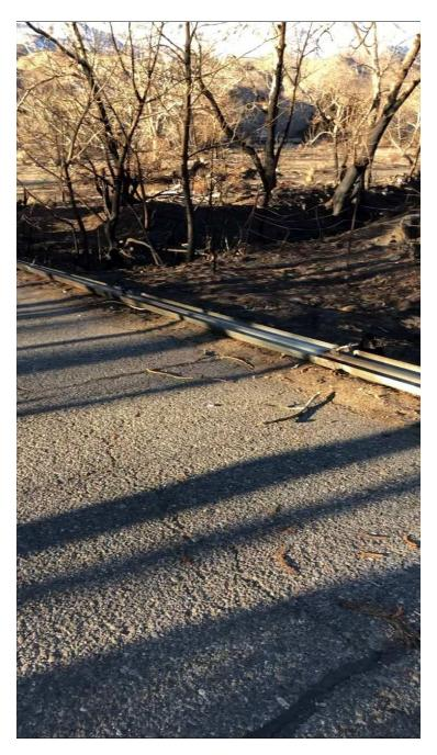
Photo 4 – North River Lane Guardrail. Westbound lane protecting from irrigation canal that crosses under road.
