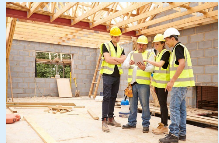
Building to higher standards prevents long-term impacts from multiple hazards, including high winds, flooding, and rising sea levels.
