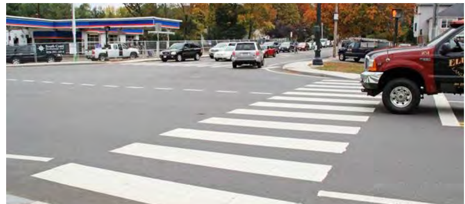
Enhances Crosswalk Markings
