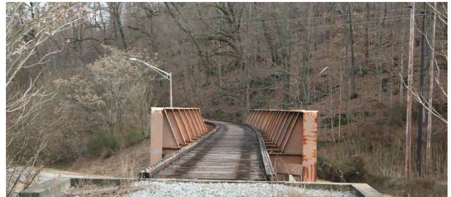
Prefabricated bridge crossings
