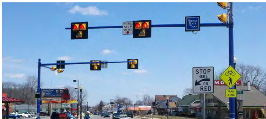
Signals and warning devices
