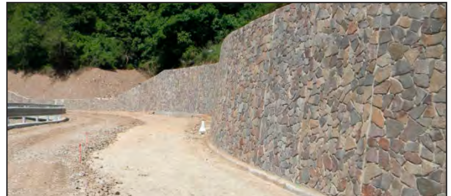
Concrete retaining walls
