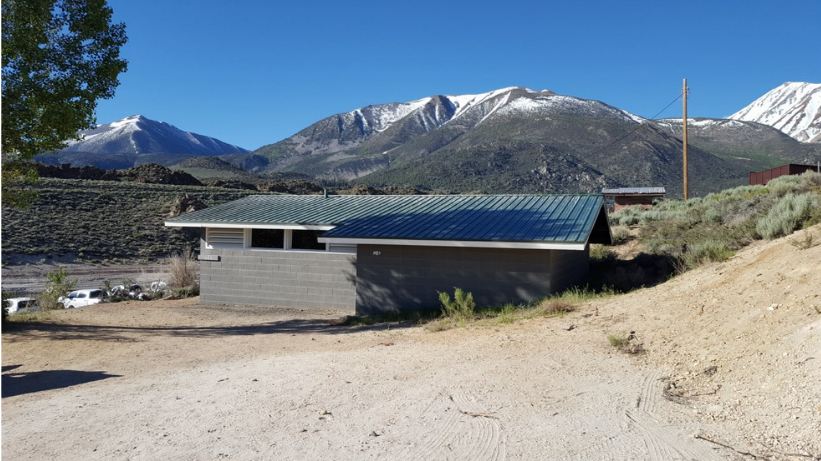
Figure 42. Public restroom, view toward south.
