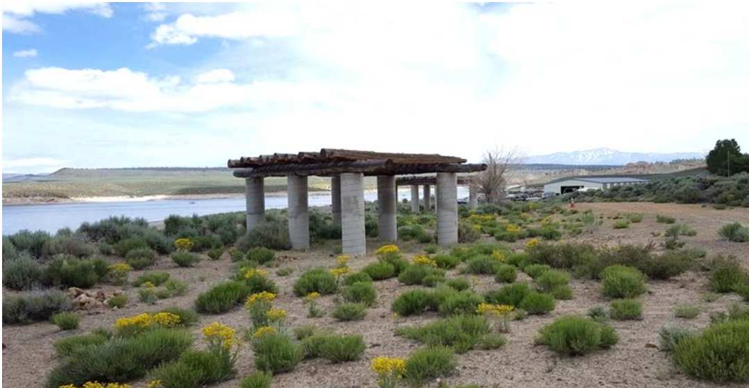
Figure 32. Ramadas, view toward northeast.
