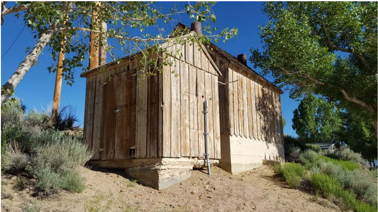
Figure 46, below. Smaller LADWP building center left, view toward northwest. Larger LADWP to right.
