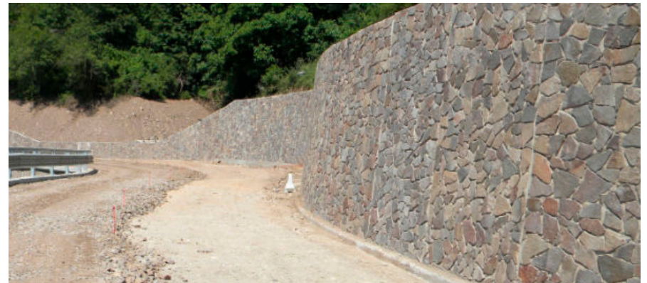
Concrete retaining walls
