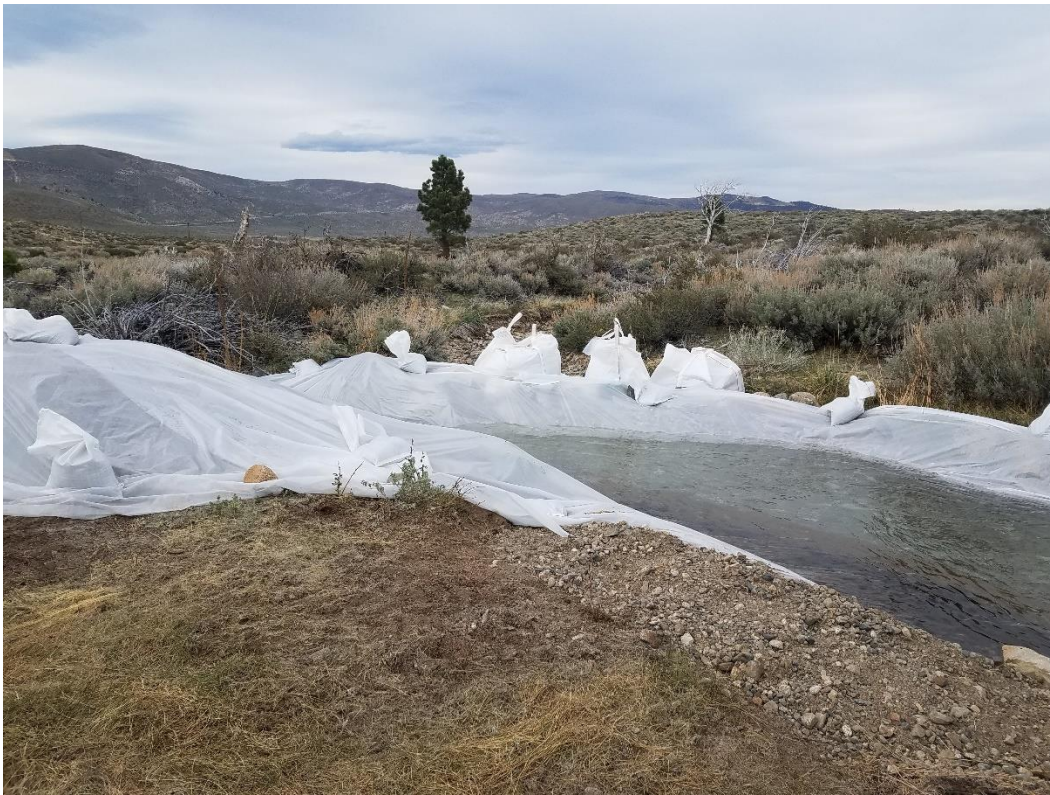
Adair Ditch Diversion Dam
