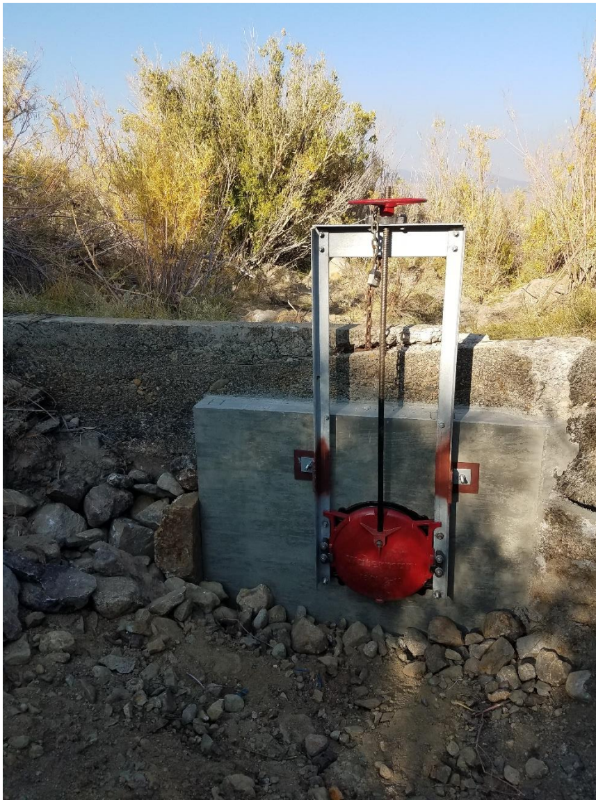
Lower Conway Ditch Head Gate
