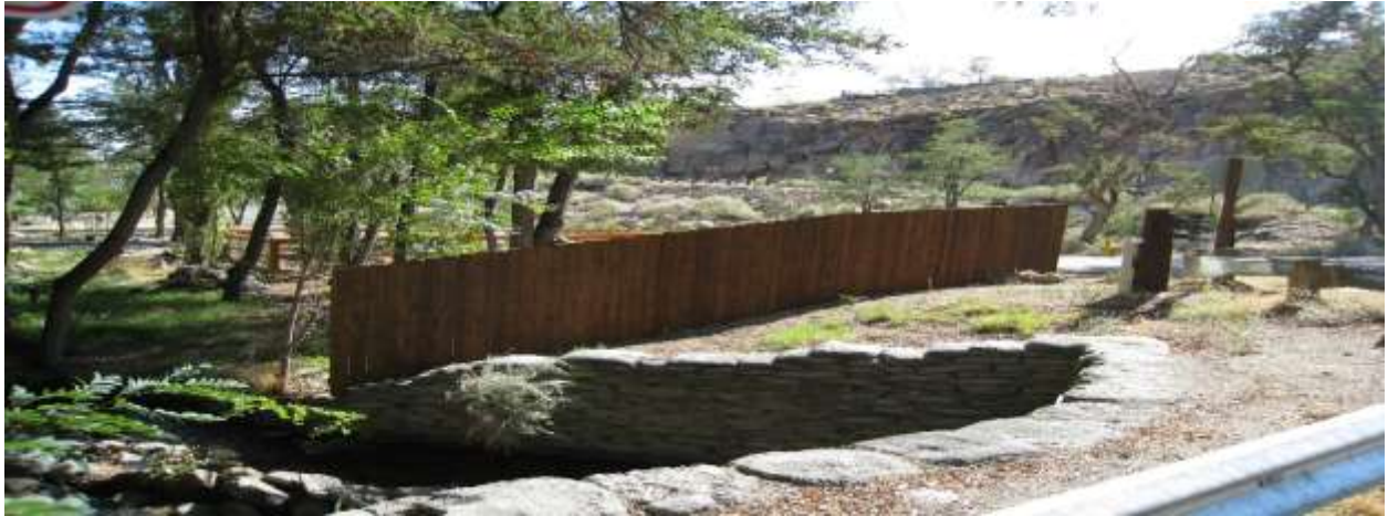
Lower Rock Creek Drive culvert bridge.
