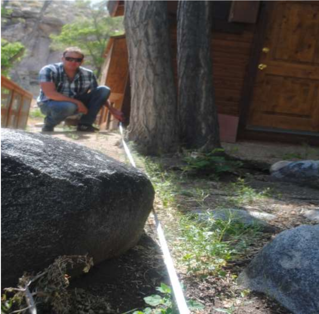
Southern corner measurement of structure corner to the irrigation ditch.
