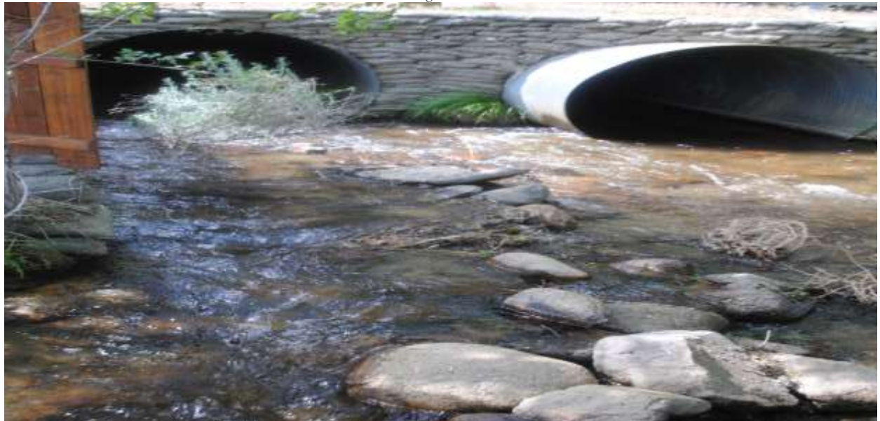
Irrigation ditch culvert and Rock Creek culvert with rock braid separation.
