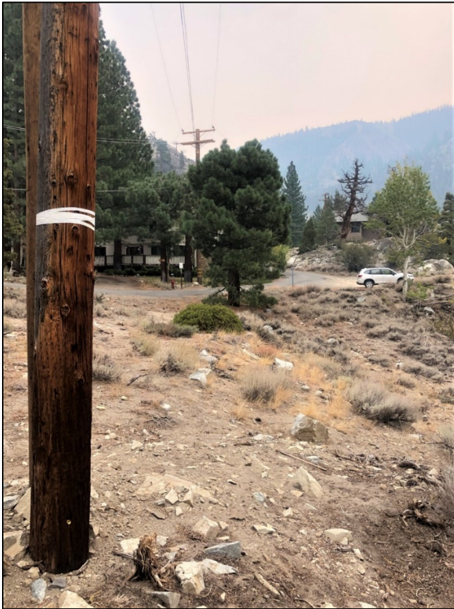
Figure 7. Southeast view of the property with SCE powerlines.
