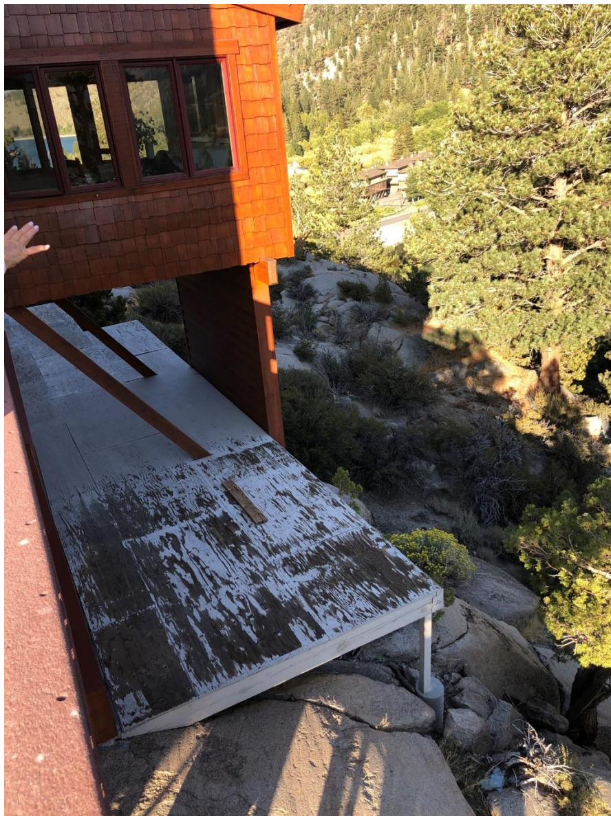
Figure 6. View from the south side of the house of the steep and rocky decline to the southeast.
