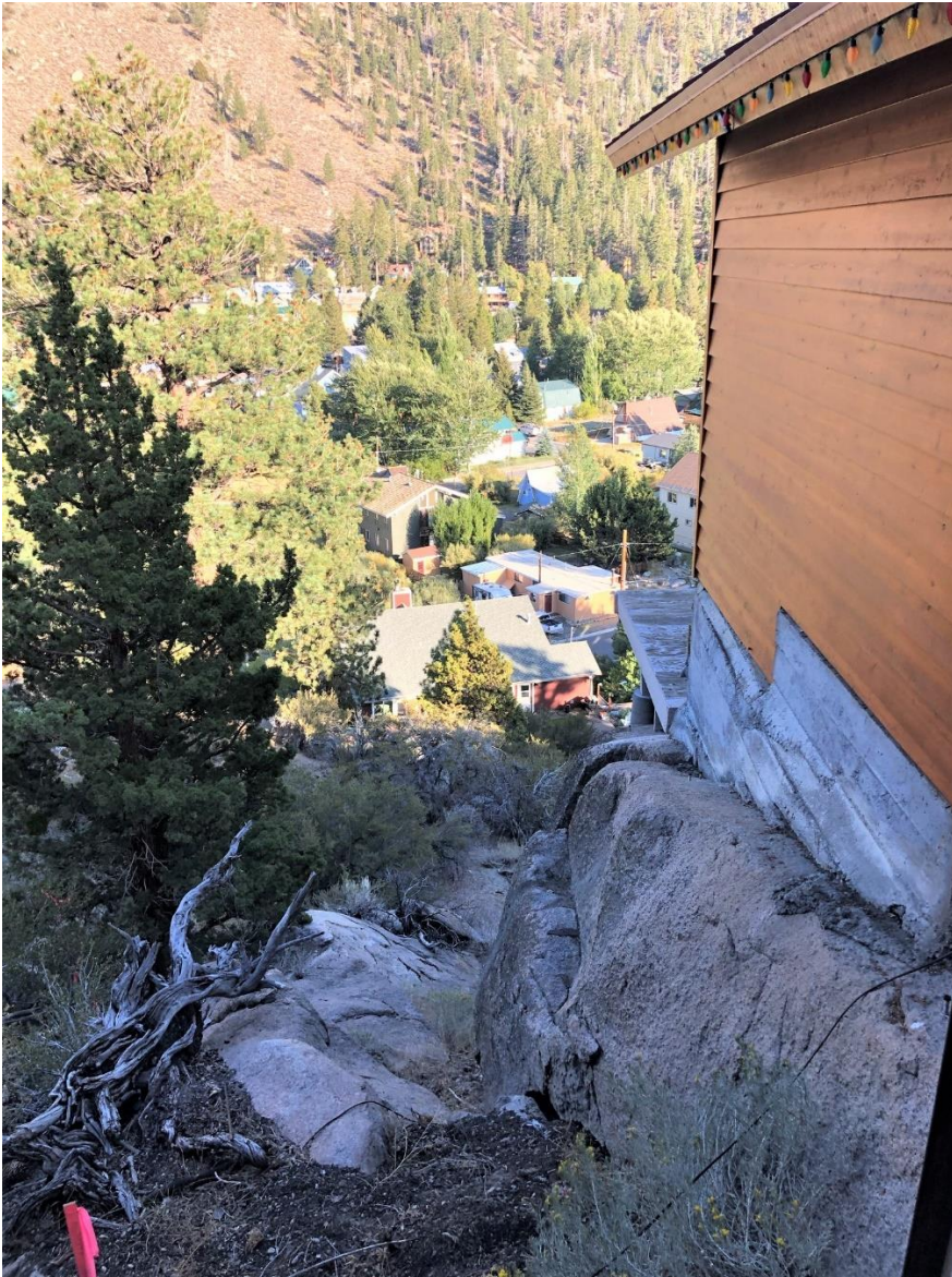
Figure 5. View along the north side of the house of the steep and rocky decline to the southeast
