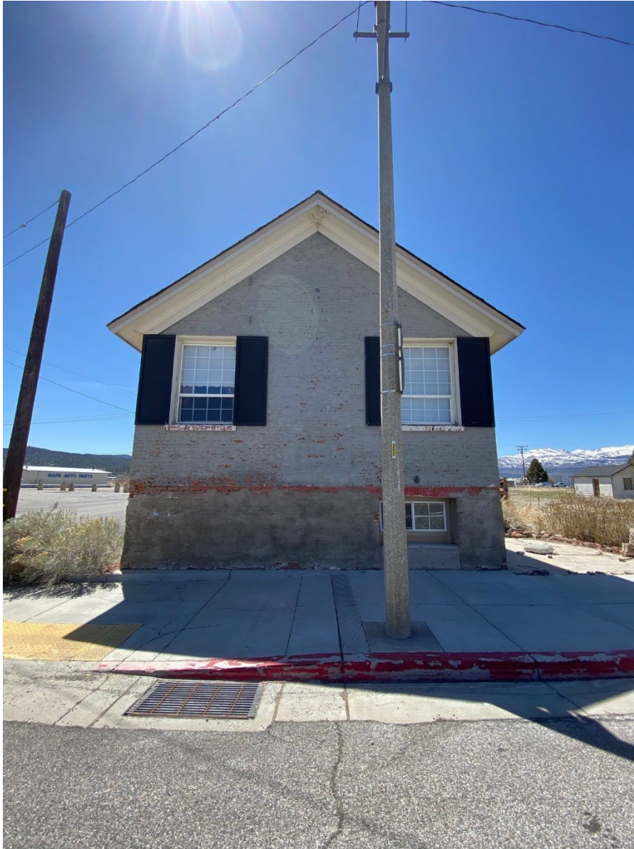
Site Photo # 1- (taken 05/04/22) View of the structure from Main Street/ Highway 395
