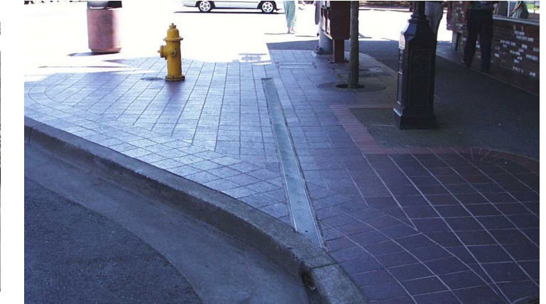
A permanent curb extension
