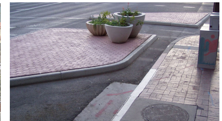
This curb extension allows water to drain to the sewer inlet, following the existing drainage line.
