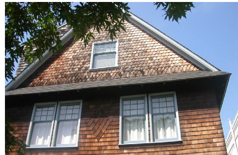
Windows are multi-paned with true or simulated muntins
